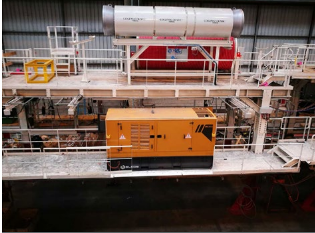
FRANCE - UNDERGROUND WORK 4 X GENSET 225/205 kVA
