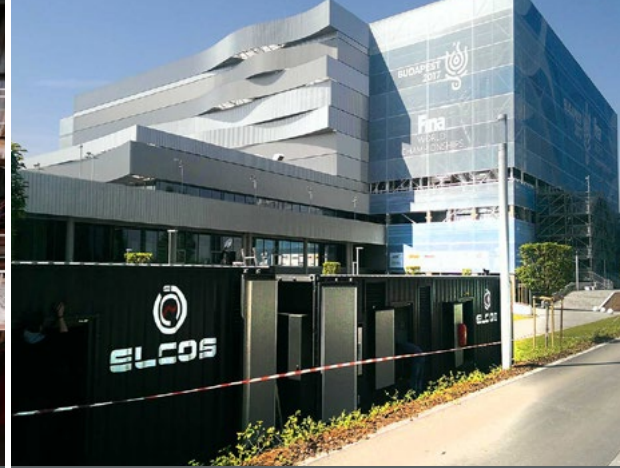
FINA HUNGARY 10 x NO BREAK Power Unit 40 kVA + 8 x NO BREAK Power Unit 20 kVA
